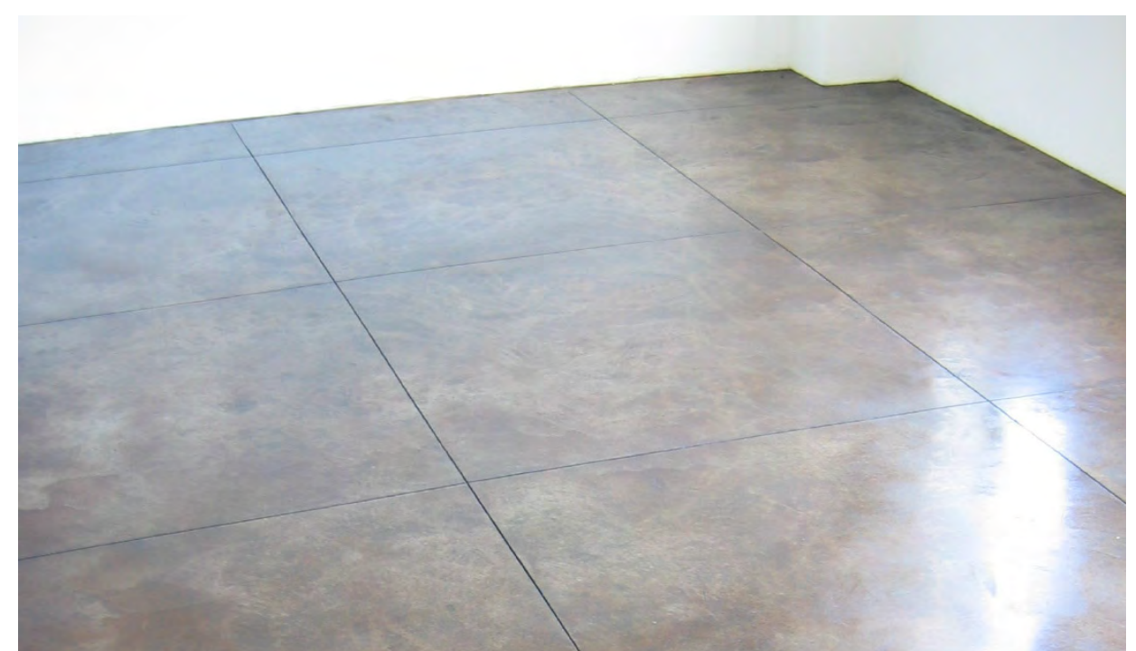
Sealed concrete is slick and can cause slipping and tripping when damp
